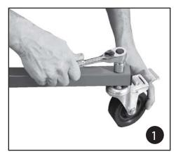
Insert wheels (9-1 & 9-2) into lower support tube (11). Tighten with wrench.
